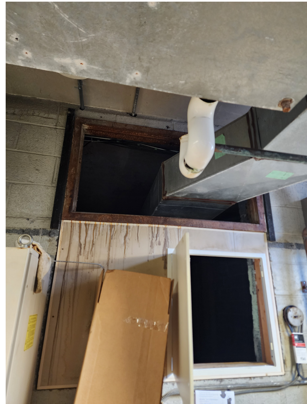
HAWTHORN HALL EXIST. ACCESS PANEL OPENING
